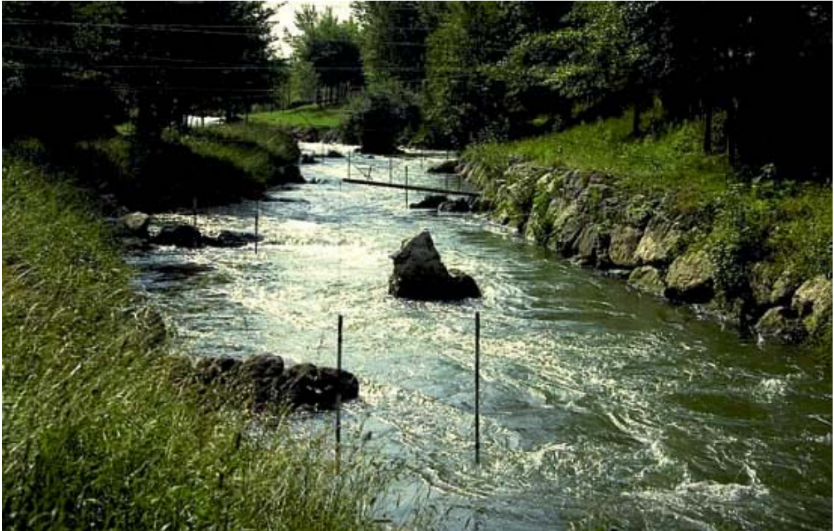
Photo 13: This natural bypass channel has been built on the Gave de Pau to overcome a 5.5 m high dam (Biron dam). The effectiveness of this fish pass has been evaluated to 100% for salmon. (Photo Larinier)
