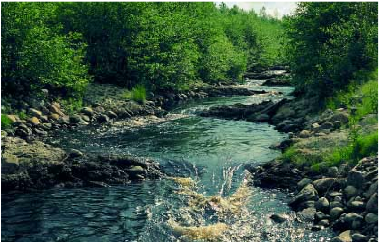
Photo 14: On the Siikajoki River (Finland), one of the fishpasses has been built as an artificial river around the dam; in 20 natural pools (with an approximate drop of \Delta h = 0,2 m between two pools) the energy is gently dissipated so that river lampreys, perch and pike can swim upstream to overcome the 4 m-high dam. (Photo Marmulla)
