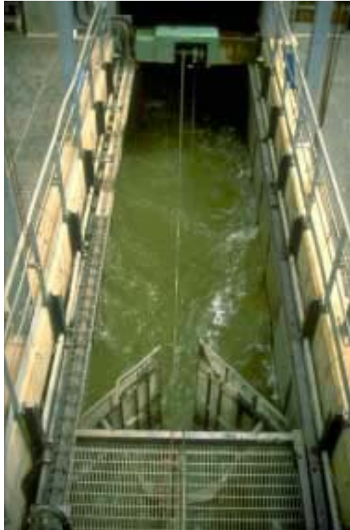
Photo 16: Holding pool and fish crowder at Golfech fish lift on the Garonne river (France). (Photo Larinier)
