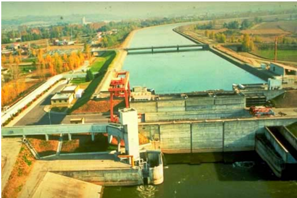
Photo 15: The fish lift at Golfech Dam ( \Delta h = 17 m) passes thousands of Allis shad ( Alosa alsosa ) each year and has thus helped to restore the shad population of the Garonne River (France) which had been cut off from valuable spawning grounds upstream. (Photo Larinier)
