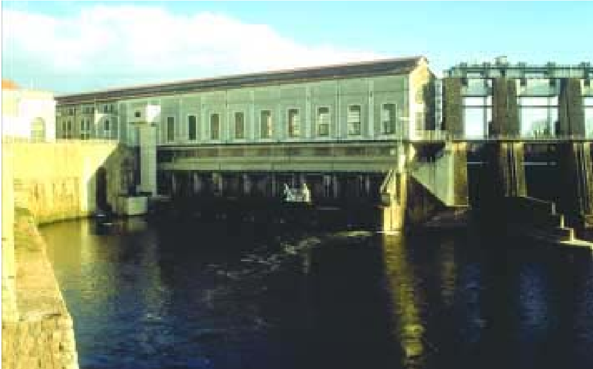
Photo 27: Due to the fish lift at the Tuilières Dam on the Dordogne River (France), migratory species such as salmon and Allis shad can now pass the obstacle and reach spawning grounds that are situated further upstream. (Photo Larinier)
