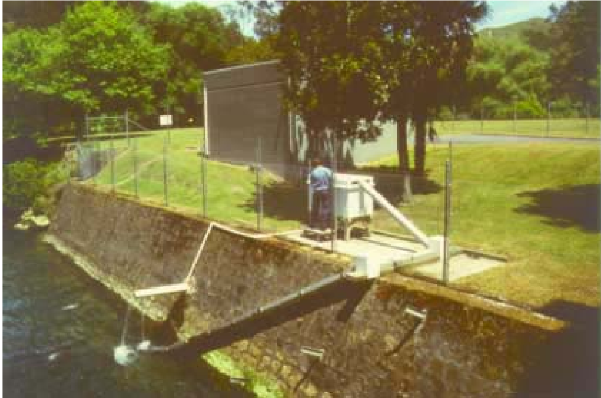
Photo 18: Young eel fish trap at Piripaua power station on the Waikaretaheke river (New Zealand). (Photo Larinier)
