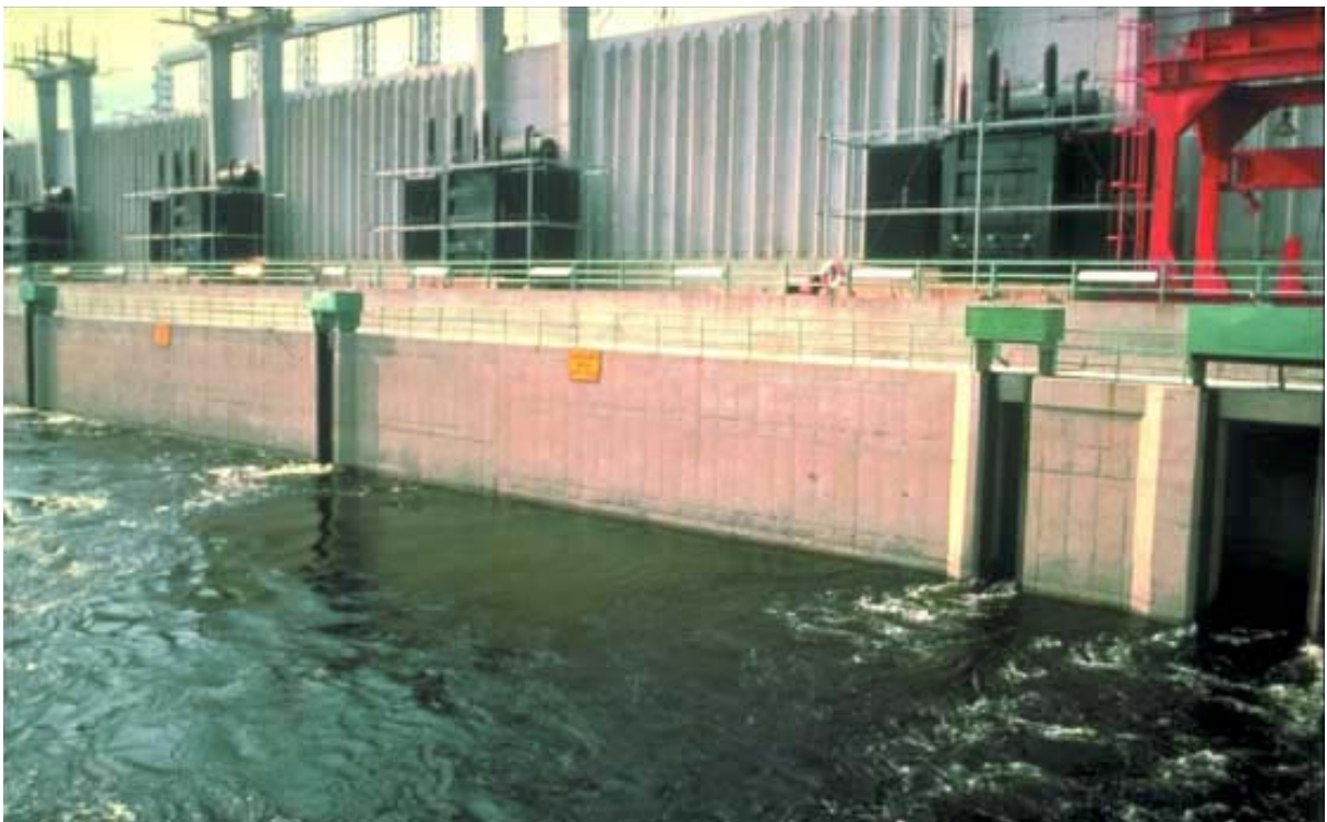
Photo 20: Collection gallery above the turbine draft tubes at Mactaquac powerhouse (Saint John river, Canada). (Photo Larinier)
