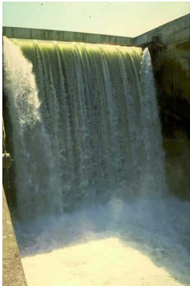
Photo 6: Spillway on the Garonne river (France).
