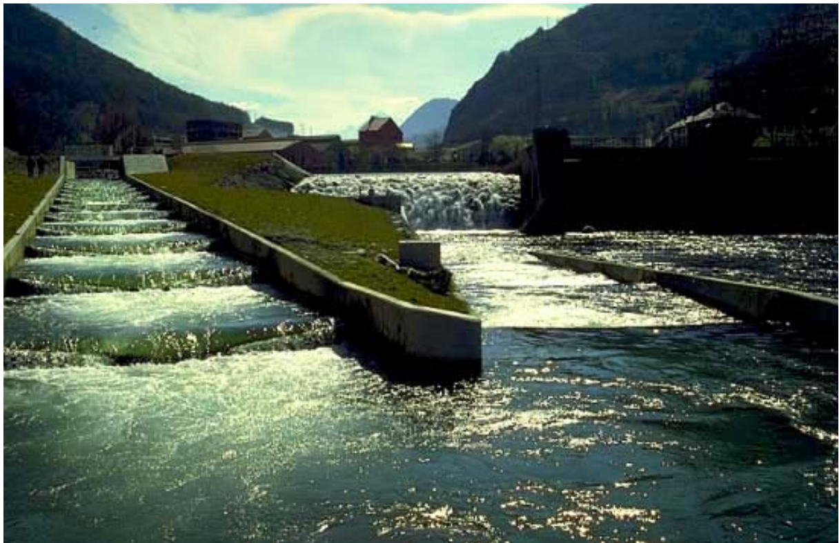
Photo 11: Pool fish pass with triangular weirs at Sarrancolin dam on the Neste River (France). (Photo Larinier)
