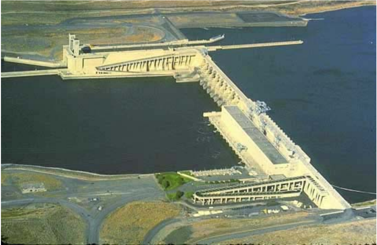
Photo 19: General view of Ice Harbor dam on the Columbia river showing the first fish pass and the collection gallery at the powerhouse and the second fish pass at the spillway. For a flow of 2800 \text{ m}^3/\text{s} in the river, the flow at the different entrances of the upstream fish facilities represents 2.6% of the river discharge (i.e. 72 \text{ m}^3/\text{s} ). (Photo Larinier)
