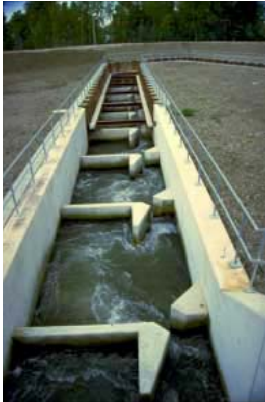
Photo 10: The fishpass at the Iffezheim Dam on the Rhine is one of the most recent vertical slot fishpasses constructed in Europe. Together with the entrance construction, the 37 pools help fish to pass the 10 m high obstacle. (Photo Larinier)
