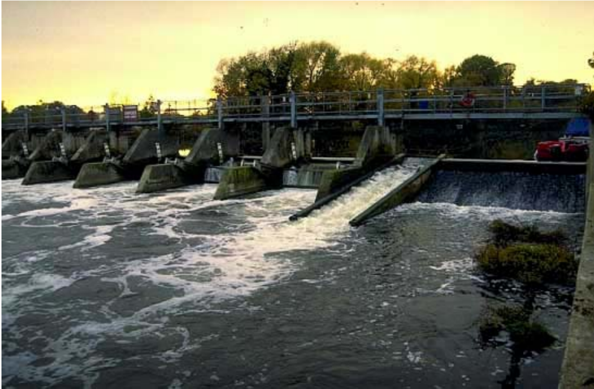
Photo 12: Floor baffles fish pass on the river Thames (UK). (Photo Larinier)
