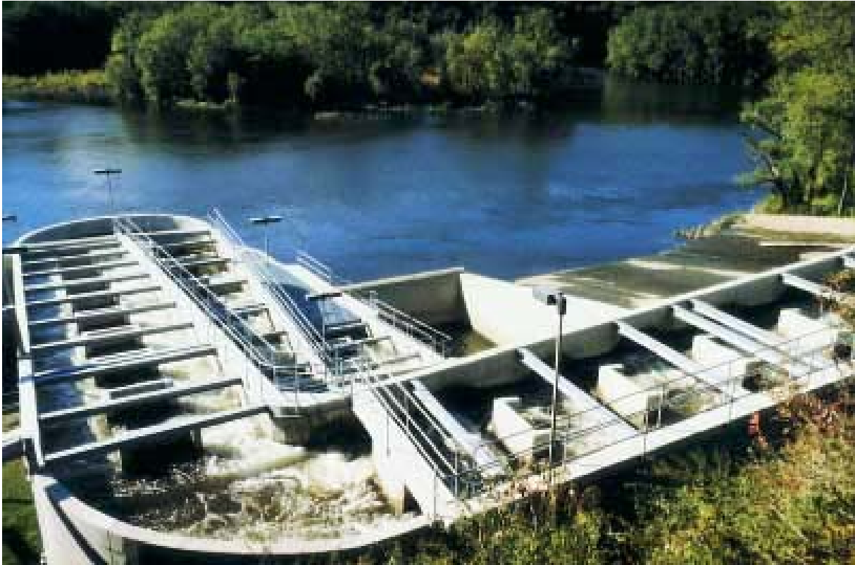
Photo 25: Ice Harbor-type pool fish pass at Turner Falls on the Connecticut River. (Photo Larinier)
