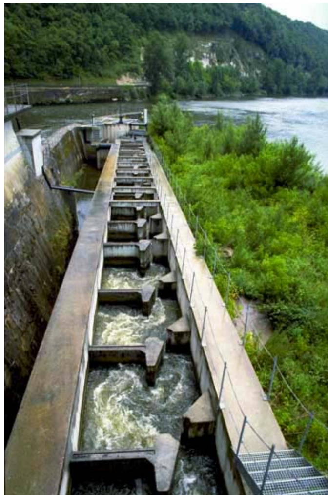
Photo 9: Vertical slot fishpass at Mauzac dam on the Dordogne River (France). (Photo Larinier)
