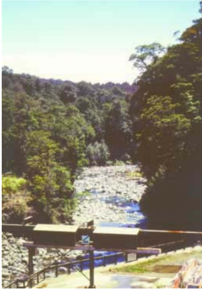
Photo 8: Drastic reduction of flow downstream a dam in New-Zealand. (Photo Larinier)
